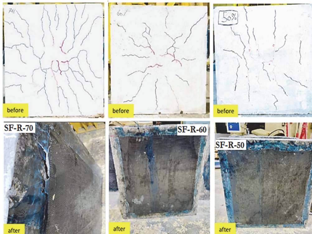
Figure 7: The mode of failure for the one layer of CFRP sheets rehabilitation technique.
