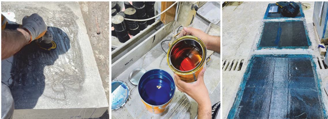
Figure 4: Mechanical repairing with CFRP sheet.
