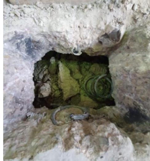
Figure 6: (S 8) After making the two holes and cutting the strand. Figure 7: A picture to illustrate the shape of the opening after casting, as well as the cut strand after tension.
