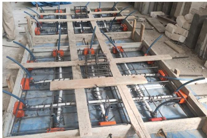
Figure 3: Details of reinforcement steel.
