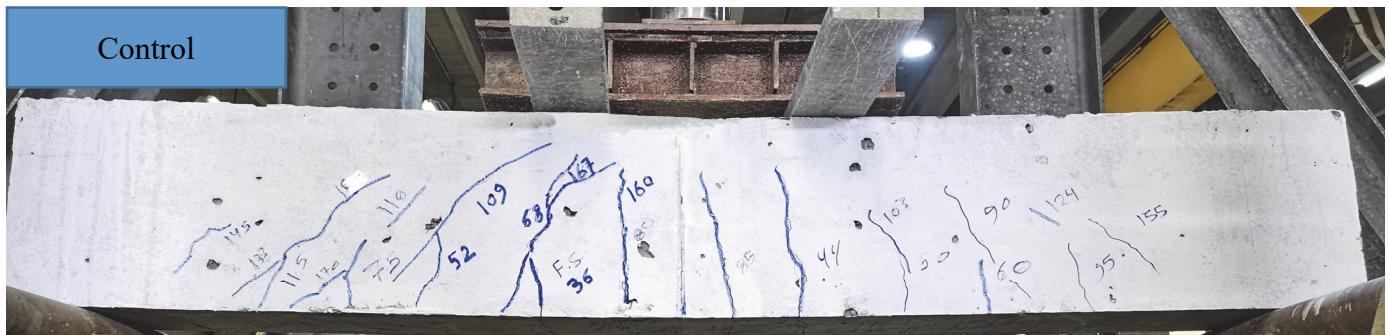
Figure 13: The mode of failure for the beam specimen (Control).
