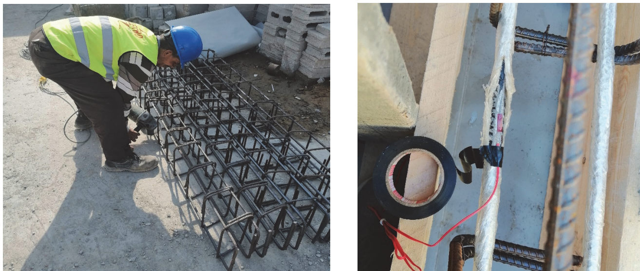
Figure 6: Installation of strain gauge and using tools.
