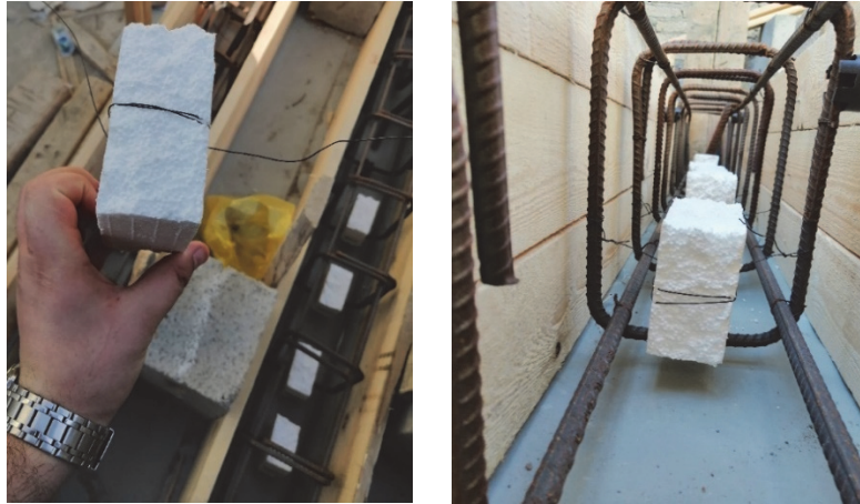
Figure 3: Overview of size and fixation of embedded foam cube.
