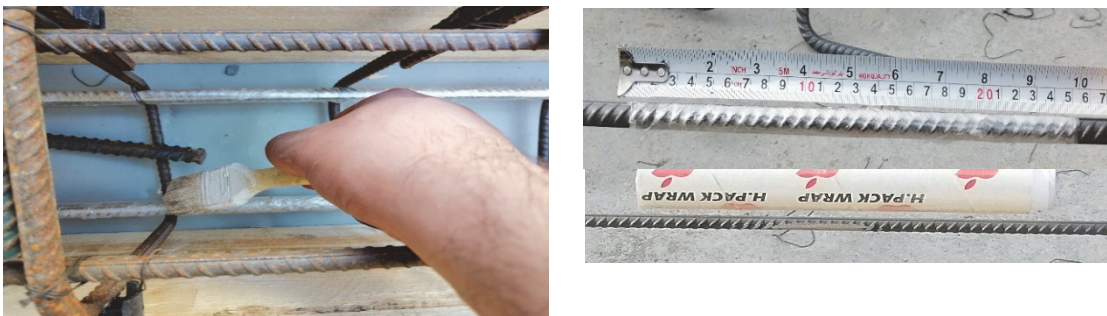
Figure 4: Process of steel isolation wrapping and painting.
