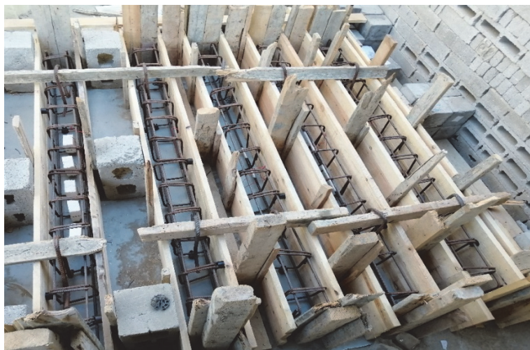
Figure 2: Wooden formwork for specimens.
