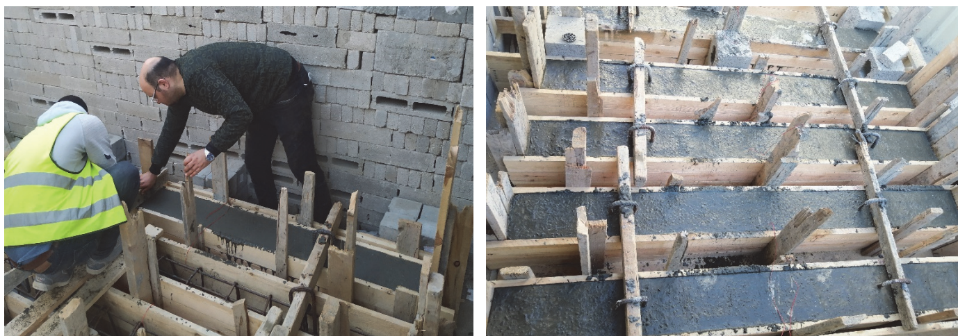
Figure 7: Beams specimens during and after casting.
