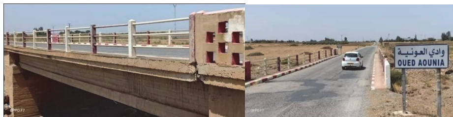
Figure 1: Oued Aounia Bridge.
