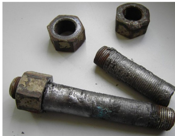
Figure 2: Clear-cut breakages of tie rods.
